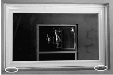
Figure 18. Water barrier method
